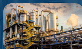
CHEMICAL & SPECIALTY CHEMICAL
